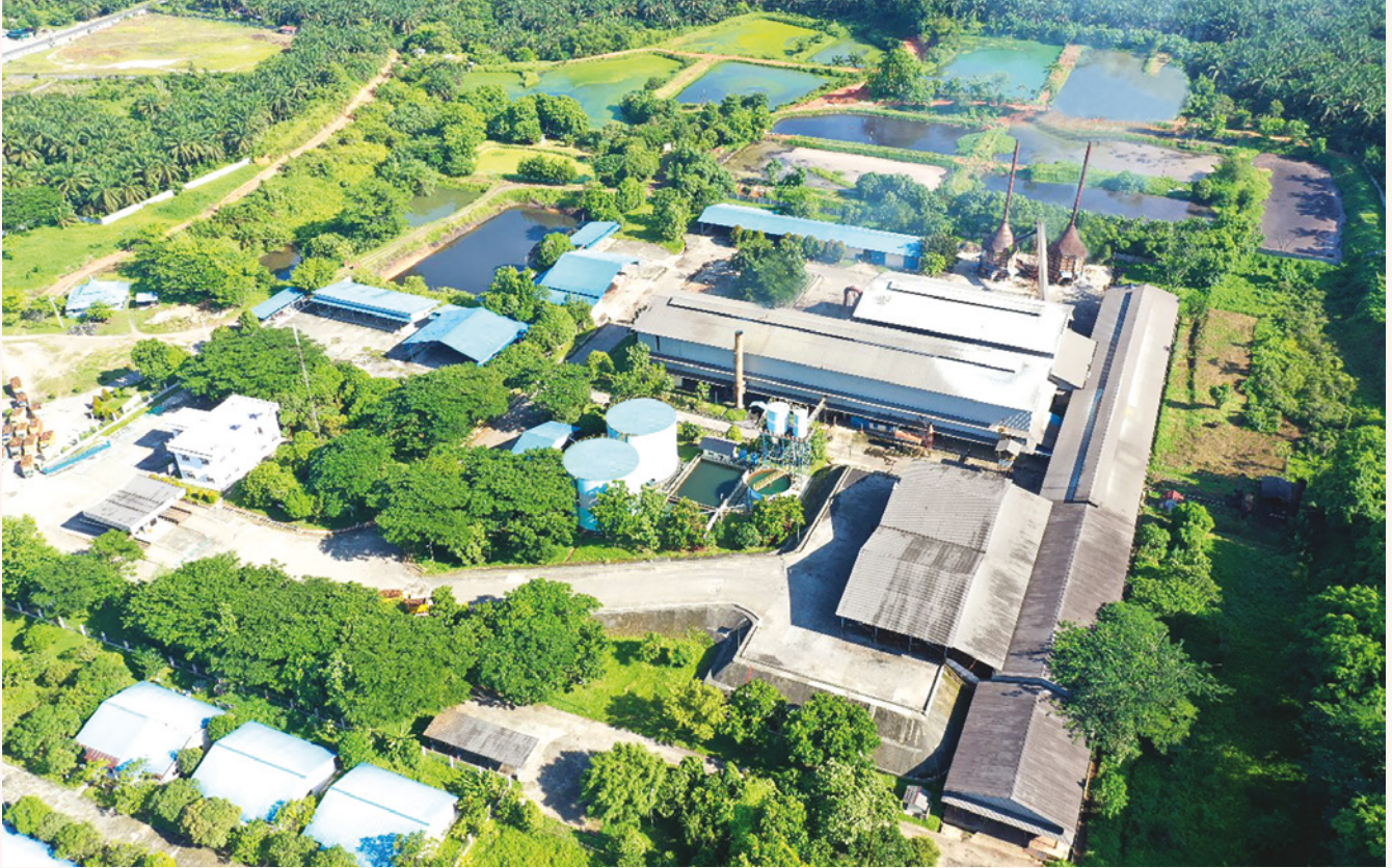
Acquired third milling plant in Riau, Indonesia on 3 April 2023.
